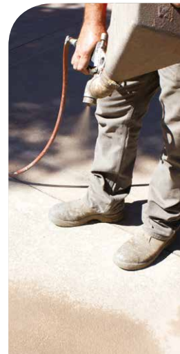
Hopper gun application of Stylepave.
